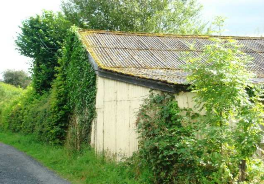
Existing corrugated buildings to be demolished
